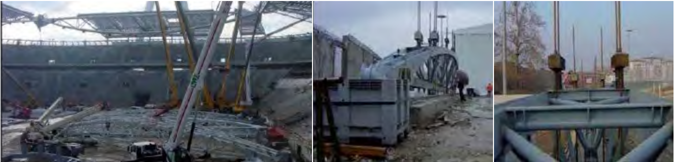
Beams tensioning of the roof of the new Juventus Stadium. Turin, Italy.
