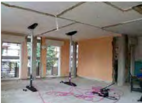
Push load test on a ceiling using COD25N260 cylinder during extraordinary maintenance works in a residential building. Milan, Italy.
